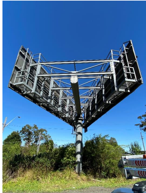
Photo 7 – General view from underside
