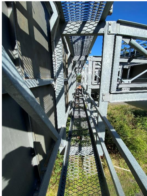
Photo 8 – General view of bottom gantry
