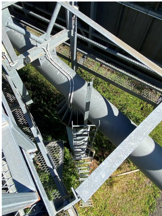
Photo 3 – Vertical access ladder viewed from above.
