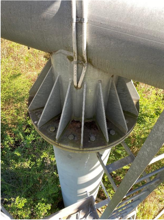
Photo 1 – Monopole to torsion beam flanged connection.
