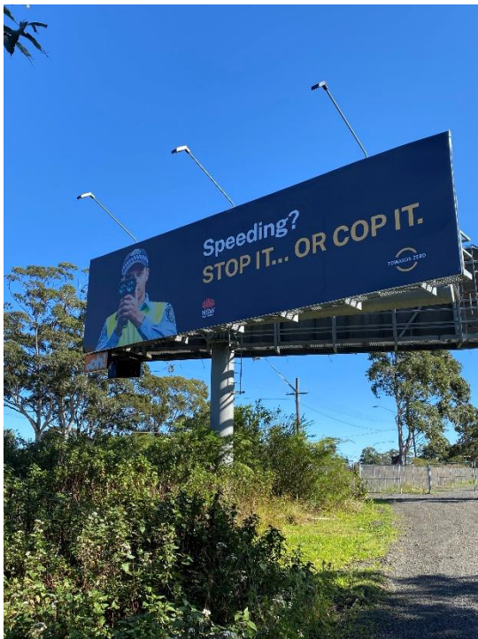
Photo 5 – General view of inbound advertising signage structure.
